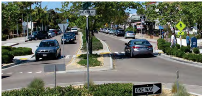
Figure 7-13: Crosswalk setback from roundabout
