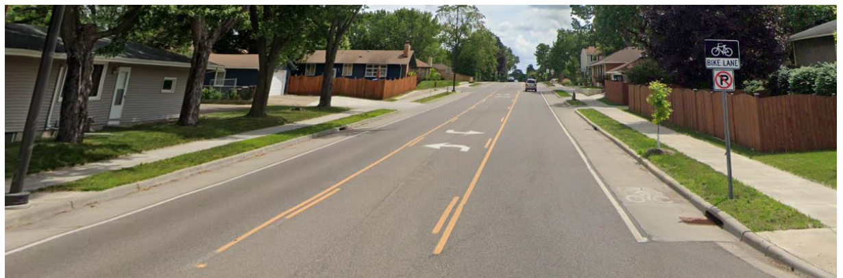
Example of 3-lane conversion with additional space allocated for bike lanes, sidewalks, and boulevard planting in Robbinsdale, MN.
