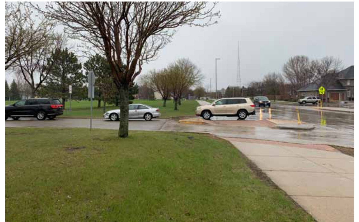
▲ Drivers blocking crosswalk; sidewalk gap along driveway; poor driving yielding and stopping compliance.
