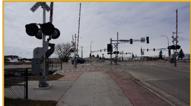
OTVR RR Crossing east of Main Avenue SE
