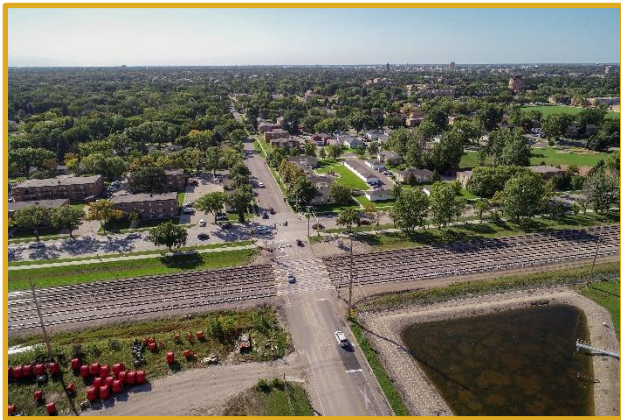
Railroad Crossing at 20 th Street
