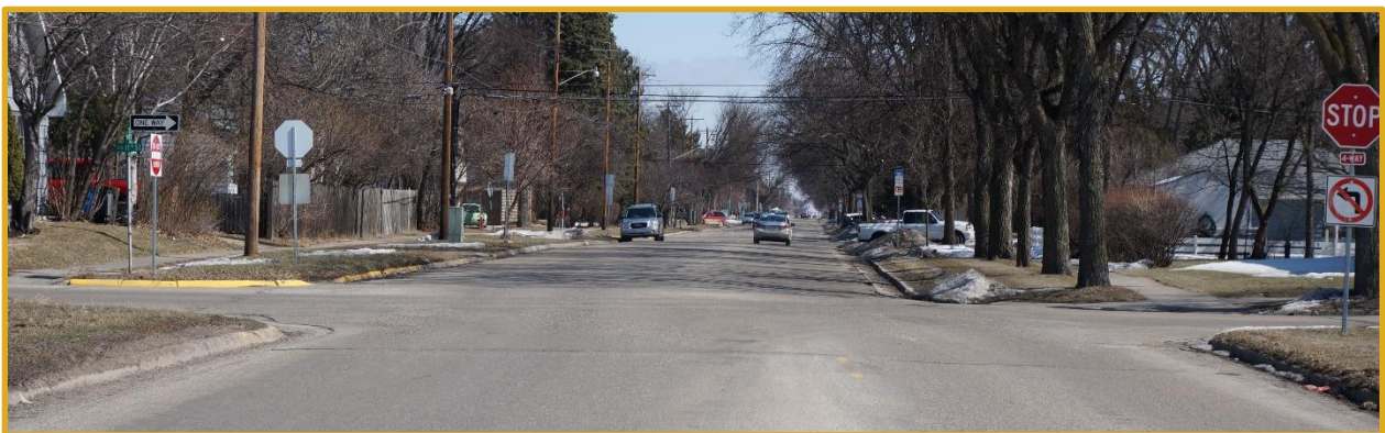
11th Street South Intersection, Facing East
