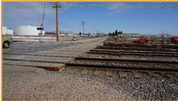
BNSF RR Crossing east of 20 th Street
