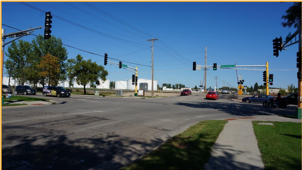
12 th Avenue and 20 th Street Intersection
