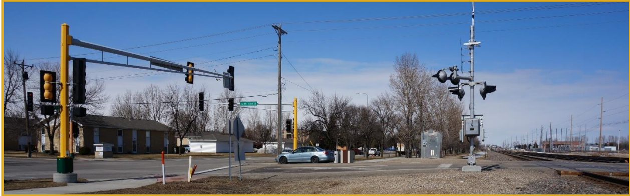
20th Street South Intersection, Facing North
