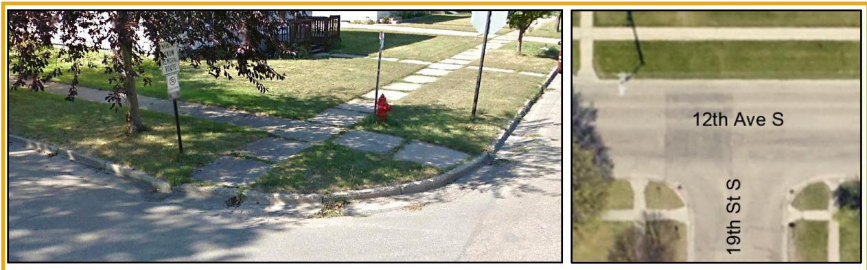
Many Sidewalk Curb Ramps Do Not Meet Current ADA Guidelines or Do Not Align
