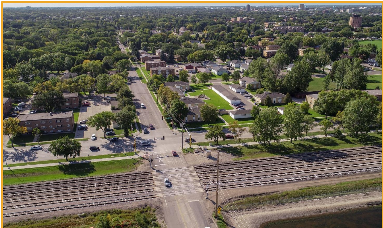
Railroad Crossing at 20 th Street
