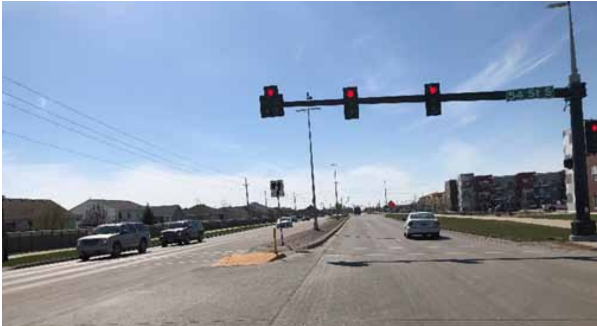
▲ The 54th Street S and 40th Avenue S intersection is very wide and lacks leading pedestrian interval to improve crossing safety.
