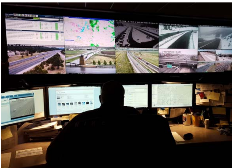
Figure 15 – Example of Traffic Operations Center Interior
