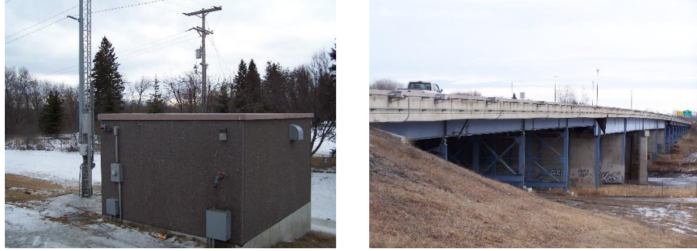
Figure 8: Red River Bridge automated anti-icing system (Source: UGPTI Site Visit)
