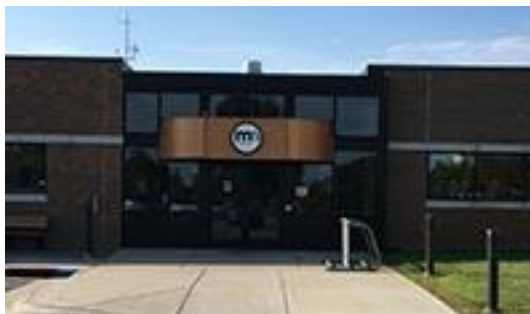
Figure 3: MnDOT District 4 Building (Source: Stakeholder)
