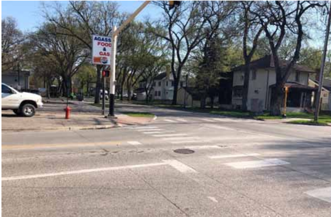
▲ Intersections with University Drive have wide curb radii and faded pavement markings.
