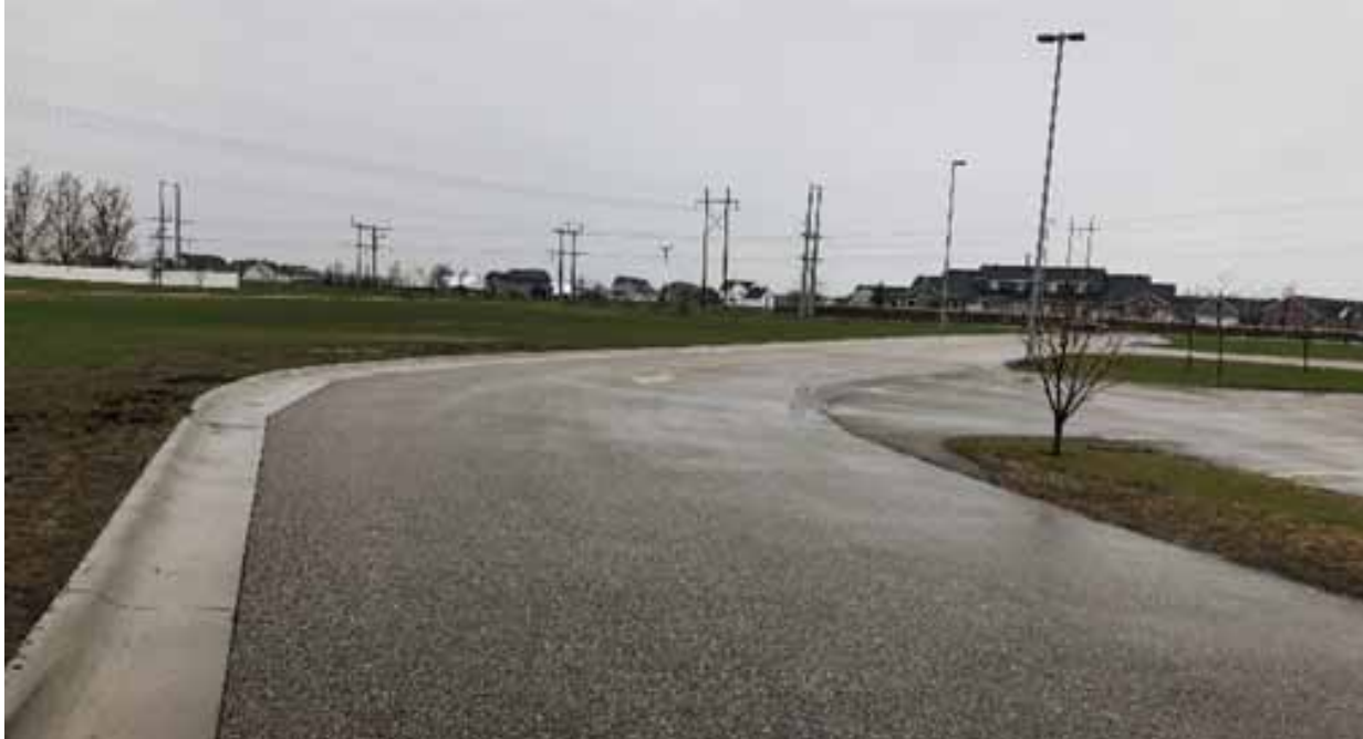
▲ There is a lack of pedestrian space around the school building and parking lots.
