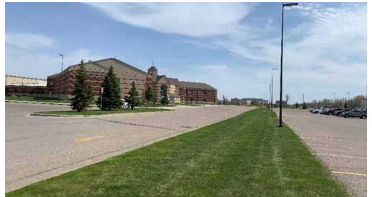
▲ Missing sidewalks along the parking lot and circulation loops.
