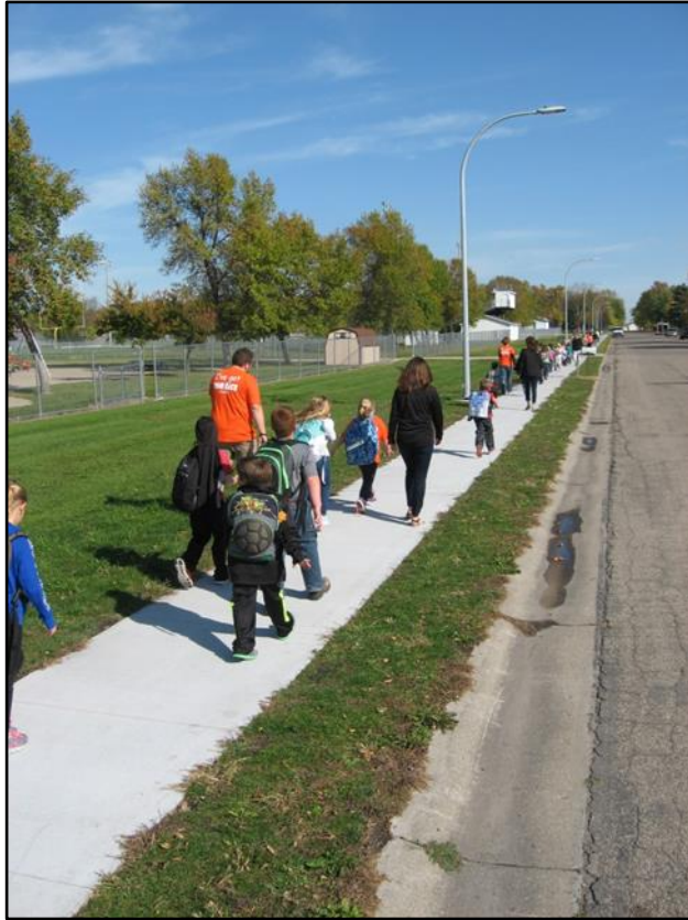
Figure 1: New sidewalks and street lights next to the Barnesville, MN football stadium were installed after the need was identified in a SRTS plan. While the sidewalk and lights were paid for with a SRTS infrastructure grant primarily to benefit students walking to and from school, these amenities are in the public right-of-way and benefit all in the community who wish or need to use them.
