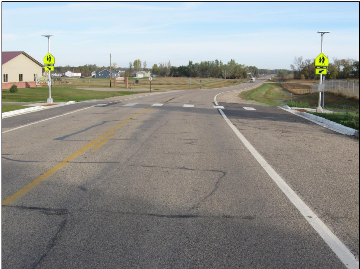
Figure 4: This crosswalk is equipped with a pedestrian (push button) activated, solar-powered Rectangular Rapid Flashing Beacon (RRFB). It is located in Frazee, MN and crosses County Road 12 near the north entrance into town. It is a prime example of an engineering SRTS solution. It was installed as part of a new trail that allows students to get to school in a more direct and safer manner. Once a pedestrian presses the button located on the sign posts, super- bright yellow LED lights flash in an eye-catching “wobble” pattern under both signs and in both directions. Otherwise, the LED lights remain turned off as seen in this photo. Driver compliance rates for crosswalks with RRFBs are significantly higher than at crosswalks without them, and can be relatively inexpensive to install.
