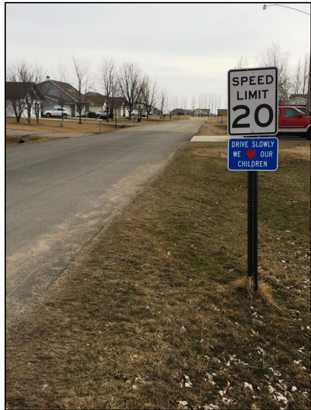
Figure 16: The 20 mph speed limit sign on Lund Ave south of 7th Street. Note the lack of sidewalks and narrow roadway.
