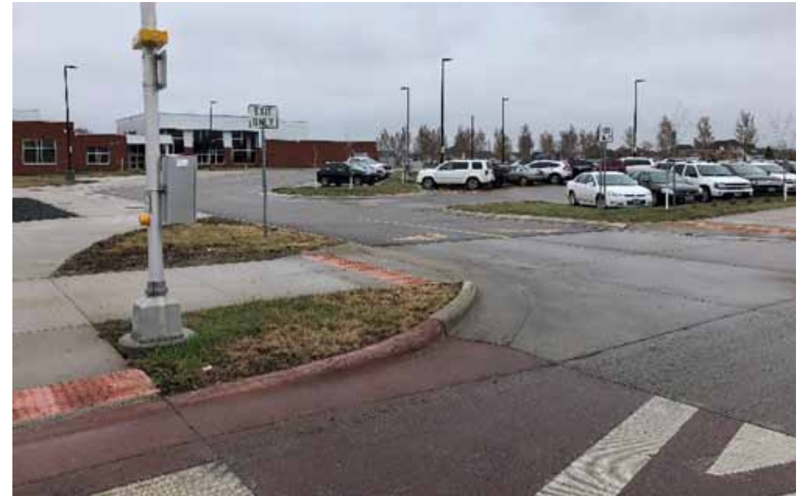
▲ Drivers do not stop or slow down when exiting driveway/turning across crosswalk. There is no signage or pavement markings.
