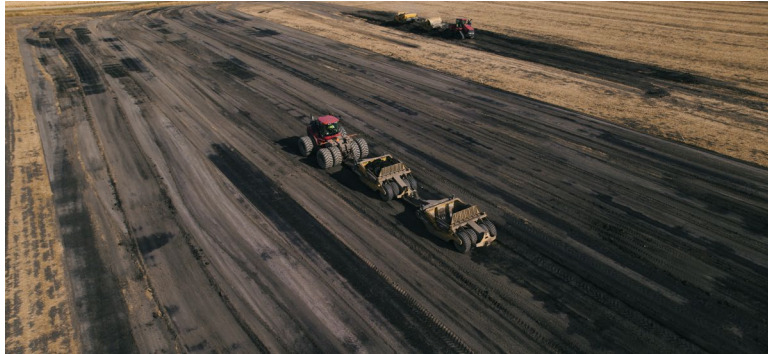
Reach 1A – 100% Completed
