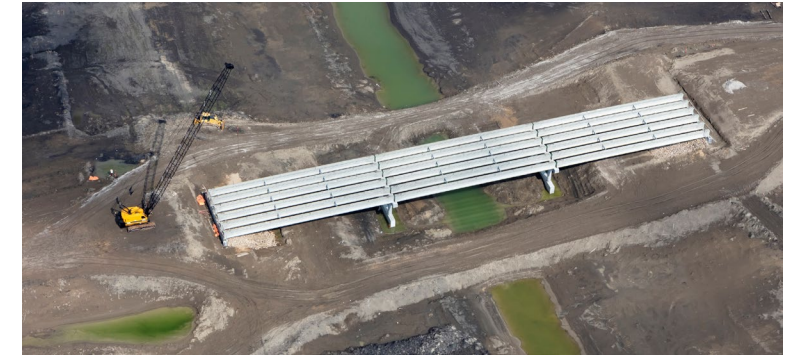
County Road - Girders
