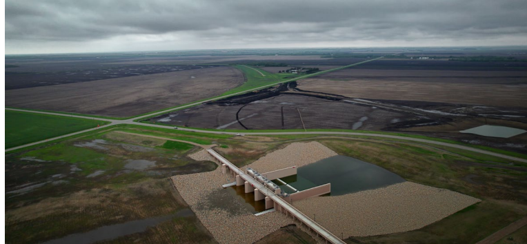
Reach 1B – 23% Completed
