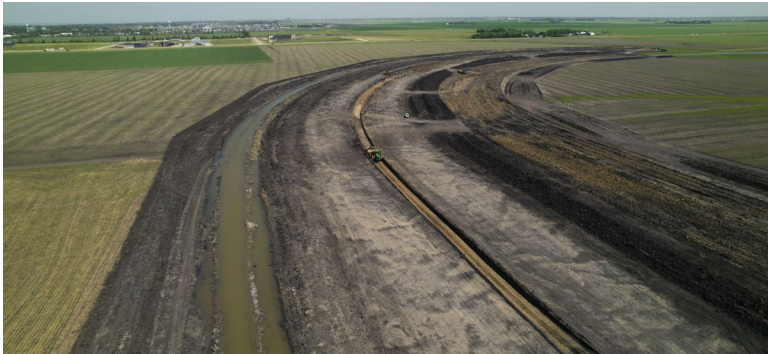
Reach 2A – 70% Completed
