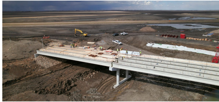
County Road - Deck Forming
