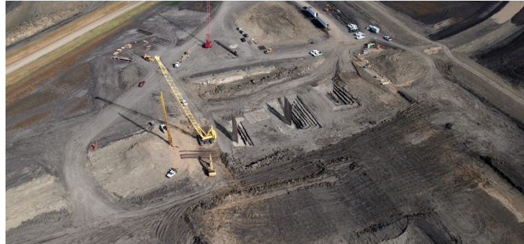
County Road - Piling
