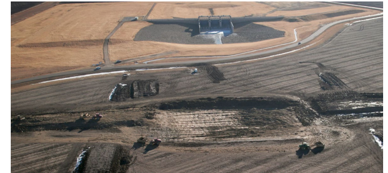
County Road - Preload
