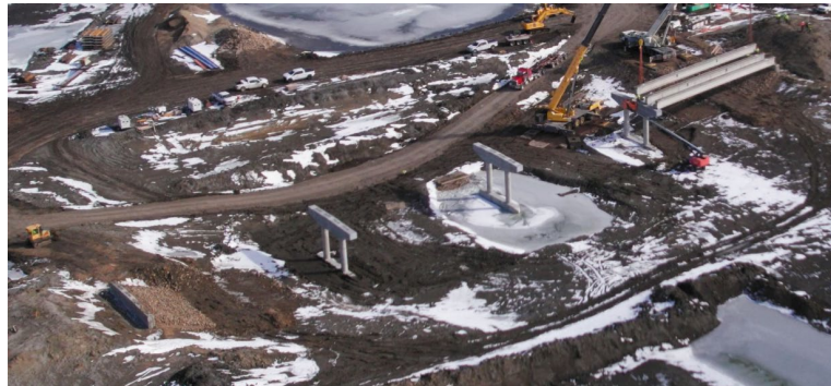
County Road - Substructures
