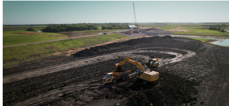
Reach 2B – 20% Completed
