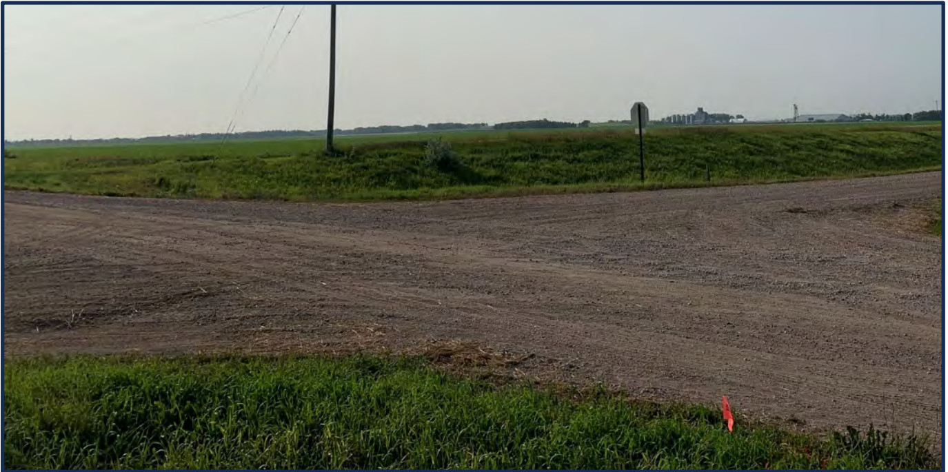
Figure 7: 15th Avenue at 60th Street looking southeast
