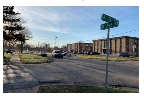
▲ Intersection is high-speed and high traffic volumes. The crosswalk markings have faded and drivers have low yielding compliance.
