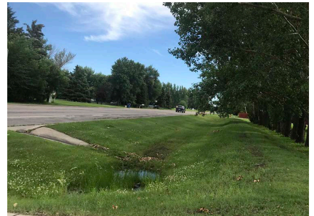
Ditches and stormwater infrastructure along the west side of 11th Street North.
