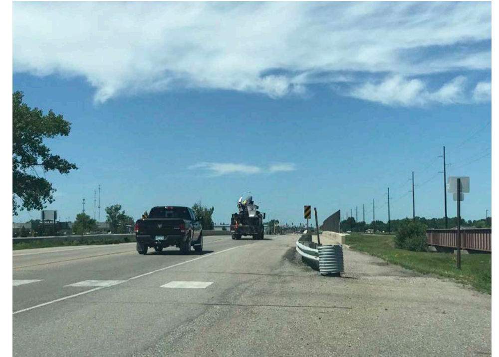
Existing conditions on CSAH 52 near 34th Street, looking north.
