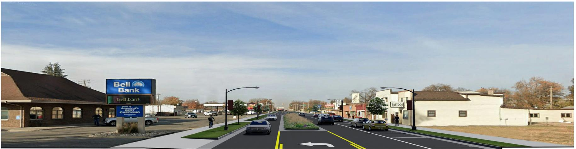
Figure 9: Highway 10 three-lane section with on-street parking
