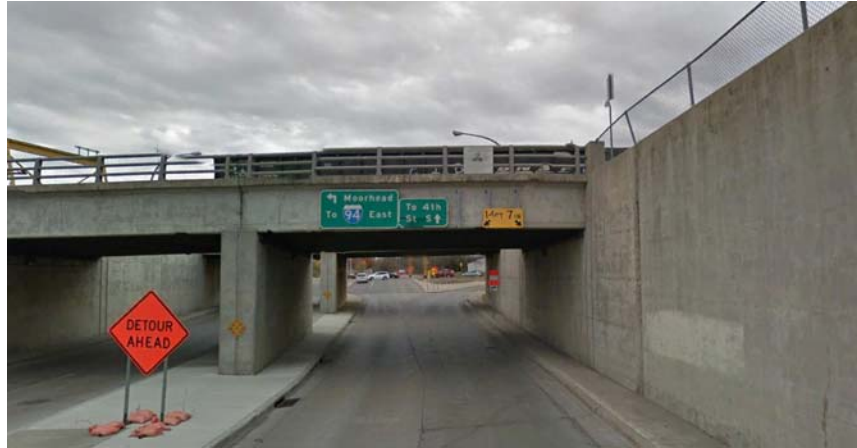
Figure 3 – Example of Low Clearance Underpass
