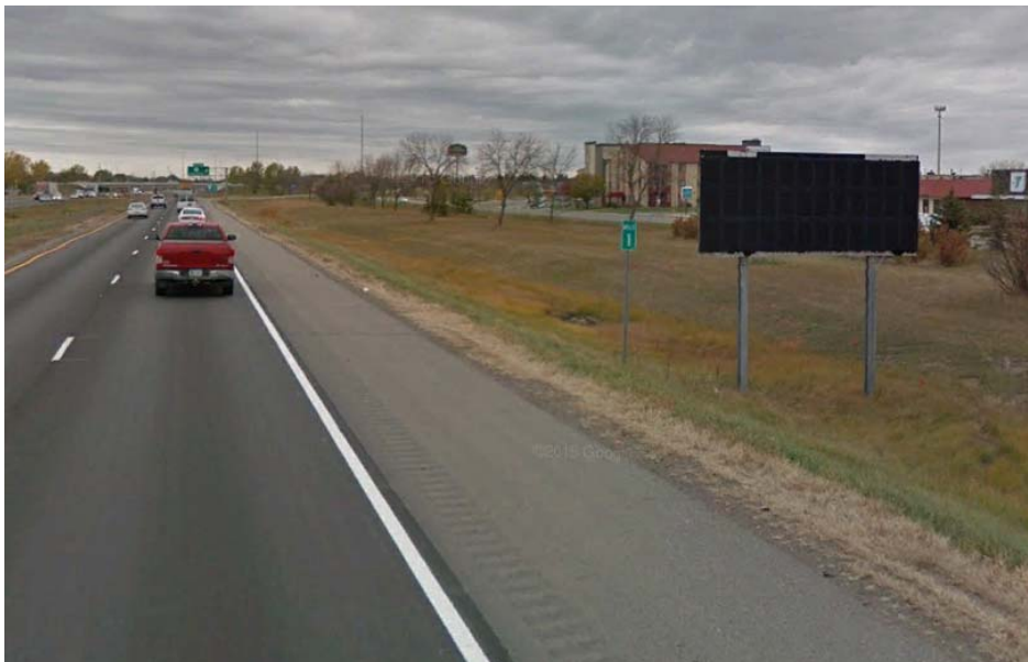
Figure 13 – Typical Minnesota DOT DMS on I-94
