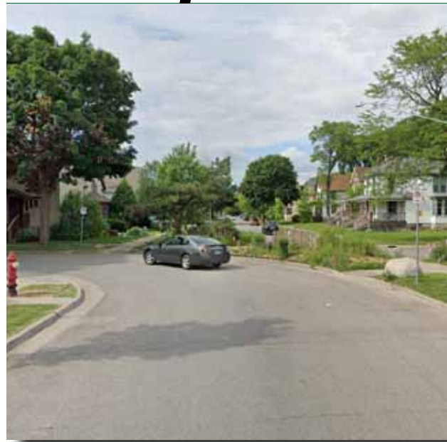
Diverter in residential area of Minneapolis, MN
