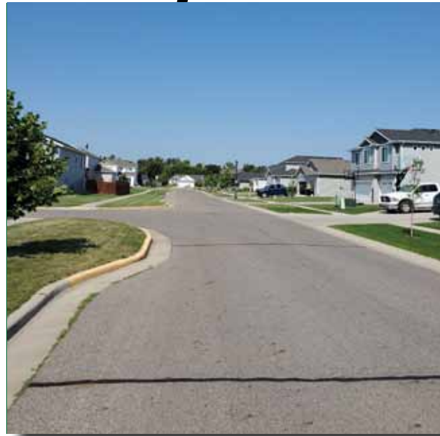
Yellow-painted curb extension narrows the roadway along 30 th Ave E in West Fargo, ND
