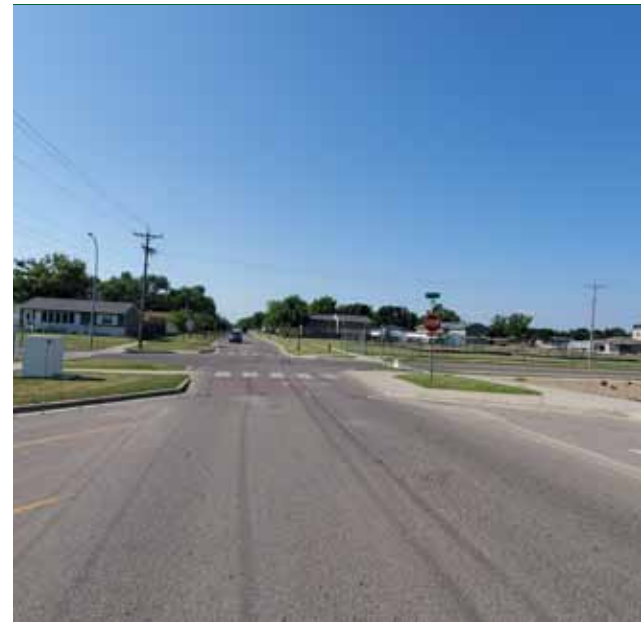
Curb extension narrows crossing of 1 st St E near South Elementary School in West Fargo, ND
