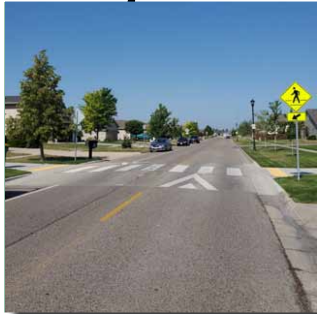
Raised crosswalk on 19 th Ave W in West Fargo, ND
