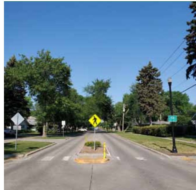
Median refuge island on 18 th Ave W in Fargo, ND
