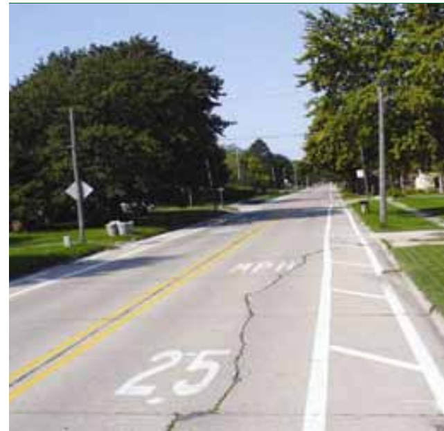
Roland, IA shoulder markings used to narrow travel lanes.
