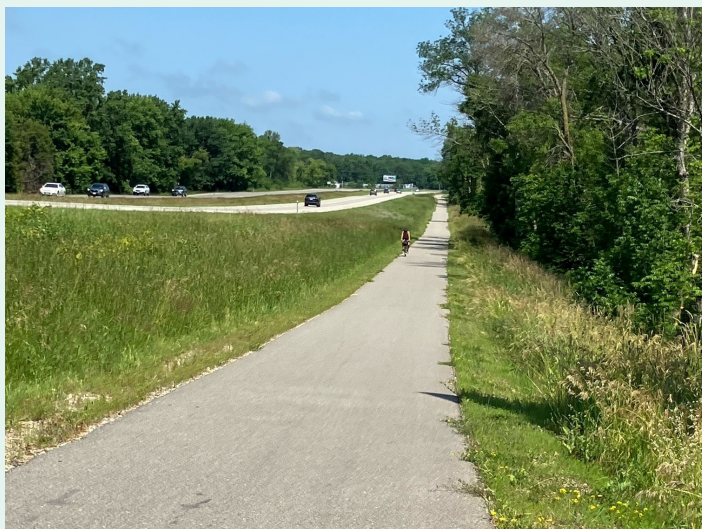
👎 Trail adjacent to HWY 10
