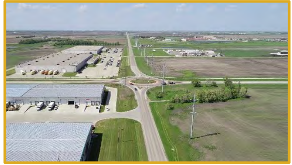
12 th Avenue Northeast – Minor Arterial
