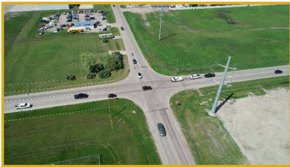
7 th Avenue Northeast – Minor Arterial
