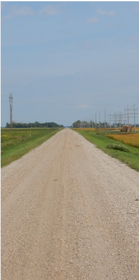
Gravel roadway between Sheyenne Street and I-29.
