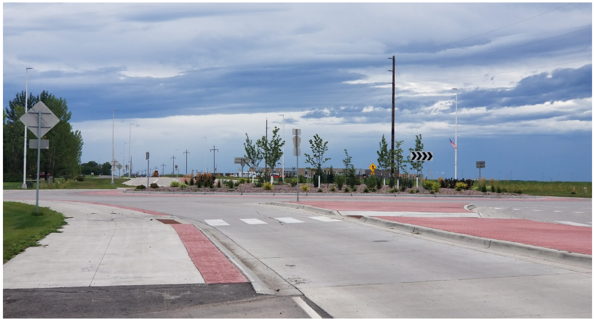
County Road 17 and 76th Avenue South Roundabout.
