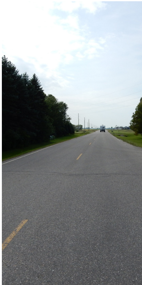
Paved roadway between 25th Street and University Drive.
