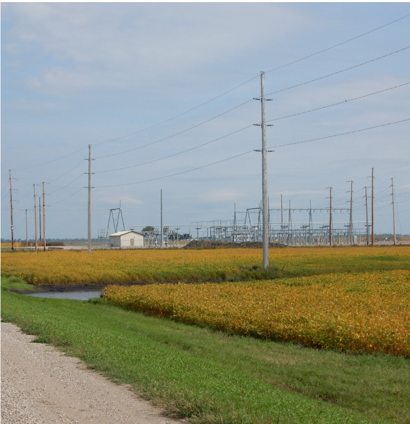
Minnkota Power overhead power lines and sub-station.
