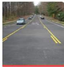
C - Undivided Roadway with Turn Lanes
