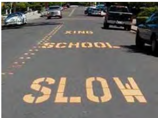
Figure 4.4 - SCHOOL XING Pavement Marking
