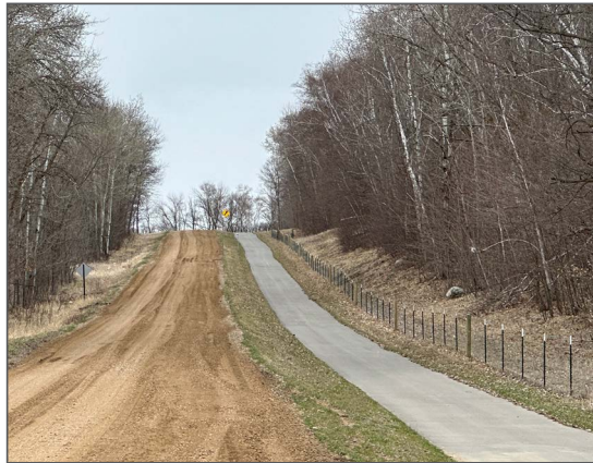
Path along a gravel road.
