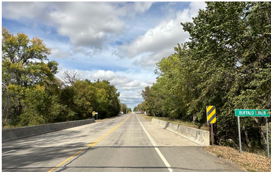
County Road 23 Bridge over the Buffalo River.
