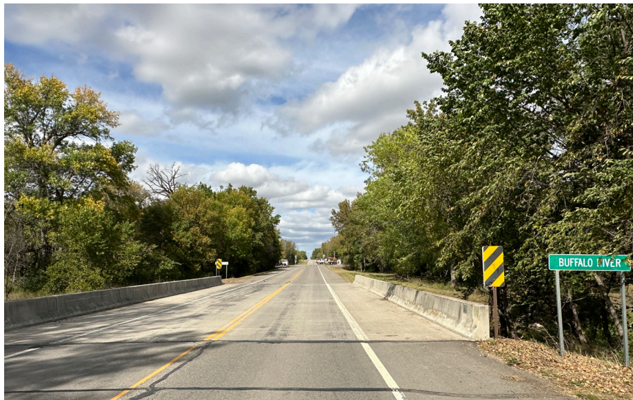
County Road 23 Bridge over the Buffalo River.
